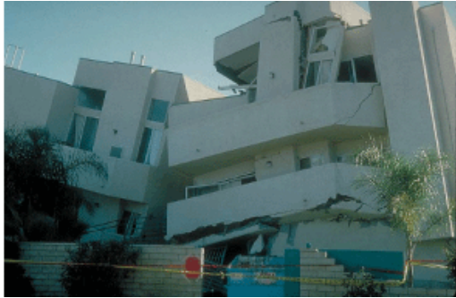
Seismic Structure response
